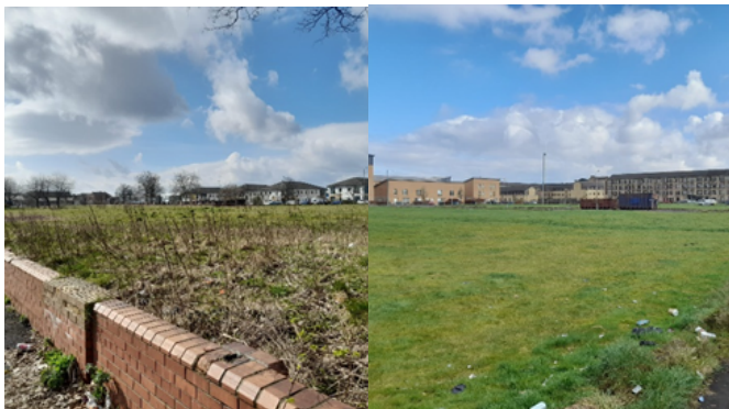
Figure: Central TRA site off Broomloan Rd where three 20-storey highrise blocks once stood (left) and the site formerly known as Iona Court (right). Photos by Gareth James.
